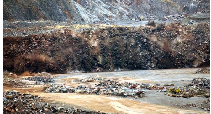
2. Blasting to break up the rock
