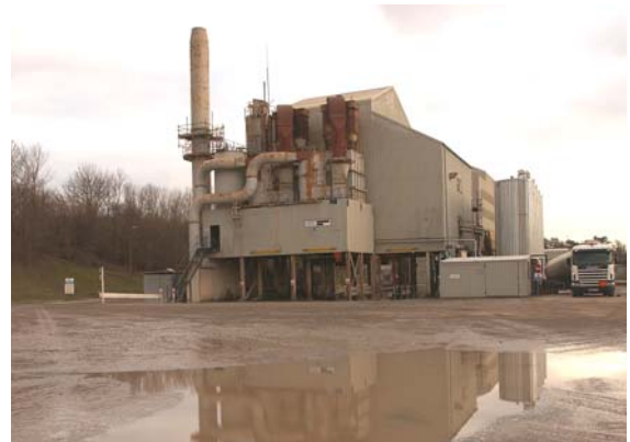
6. Producing asphalt for roads
