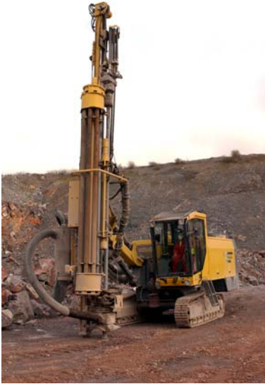
1. Drilling the rock-face
