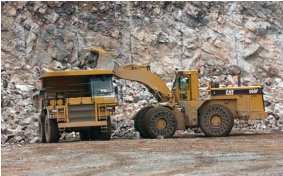
3. Loading dumper at rockface
